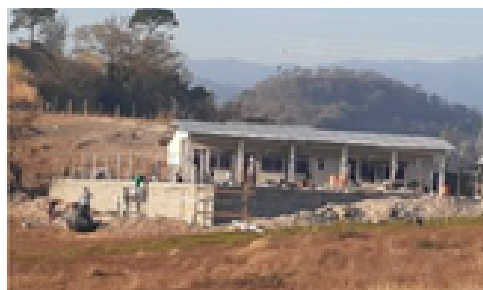
Retaining Wall Implemented in 2020
